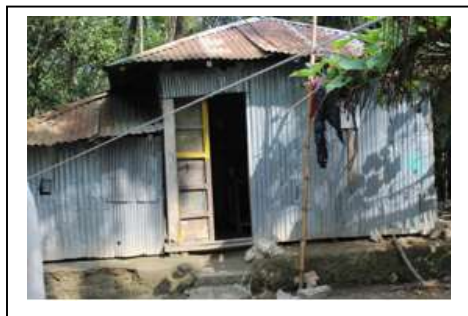
A CV House provided by CDSP I
